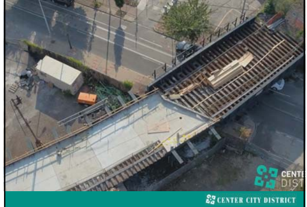
Renovated bridges, poured new concrete slab
