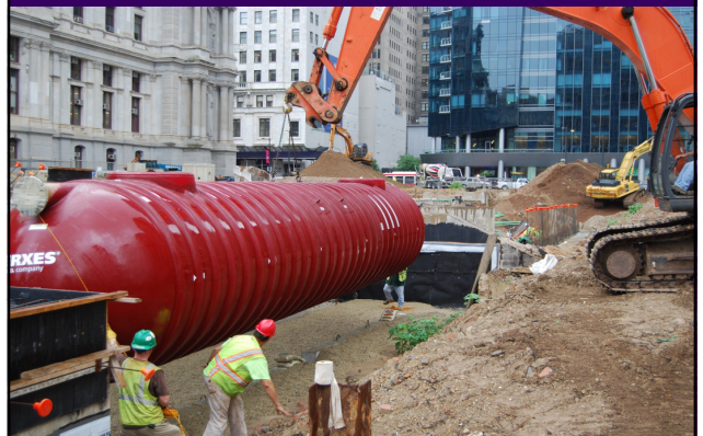
Storage tanks for installed during construction
